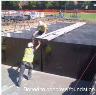
3. Bolted to concrete foundation
