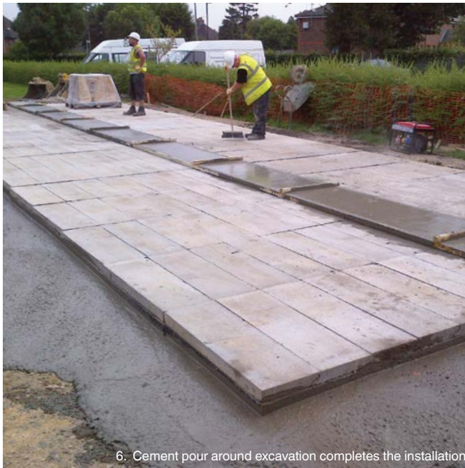
6. Cement pour around excavation completes the installation
