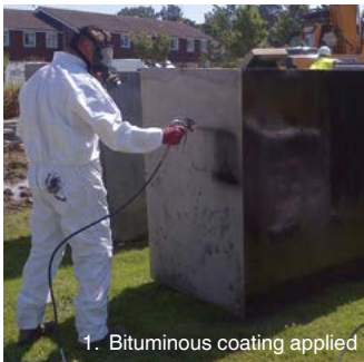
1. Bituminous coating applied
