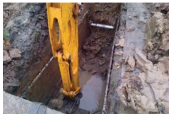
Excavating earthen graves in wet ground can be dangerous and risk of grave collapse is high.
