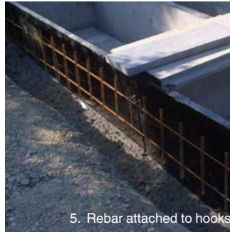
5. Rebar attached to hooks
